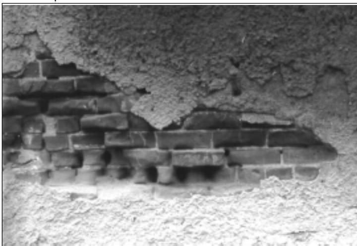
Surface coating that traps moisture can cause extensive damage to masonry.
