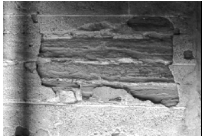
Stucco applied to limestone has trapped moisture in the wall. Freezing caused the stucco to loosen and break away, taking bits of the stone with it.
