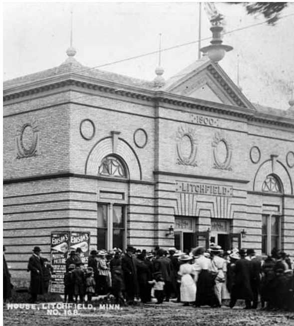
Litchfield Opera House, 1908, MHS Photograph Collection
